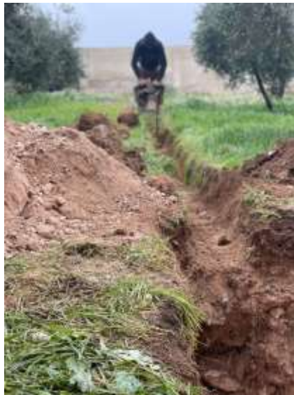
Figure A.1 Excavation work
