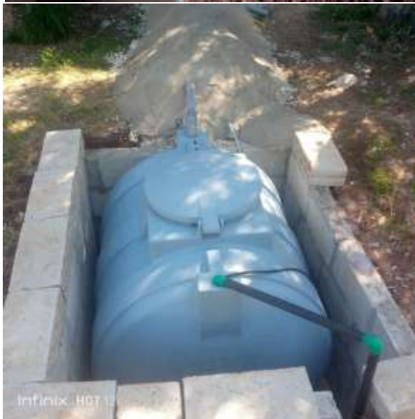
Figure A.10 Tanks installation
