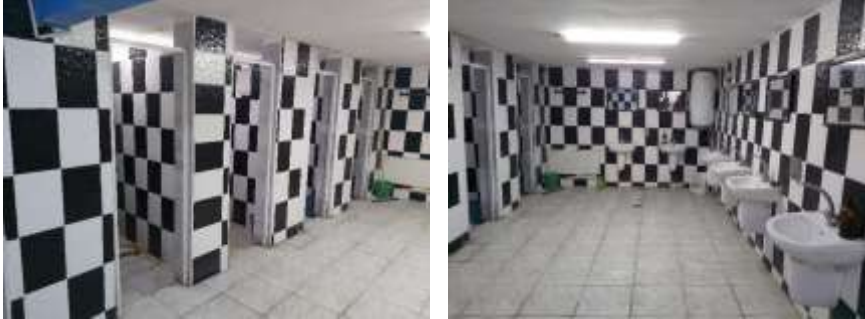
Figure 3 WASH unit – ablution area
