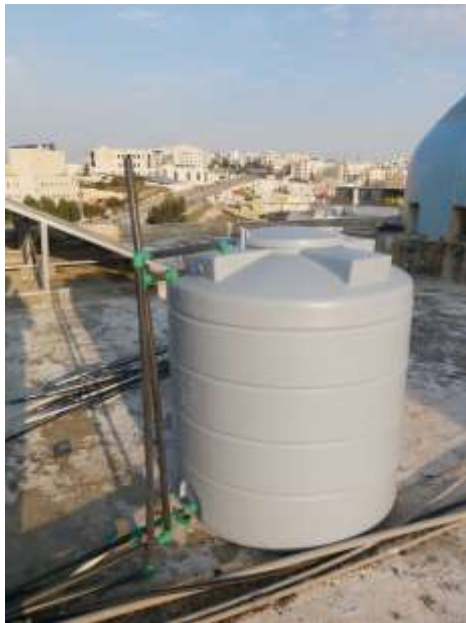
Figure A.8 Roof tank for irrigation
