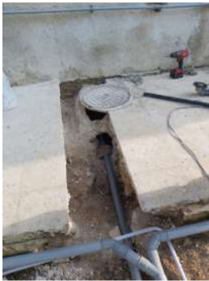
Figure A.3 Plumbing works
