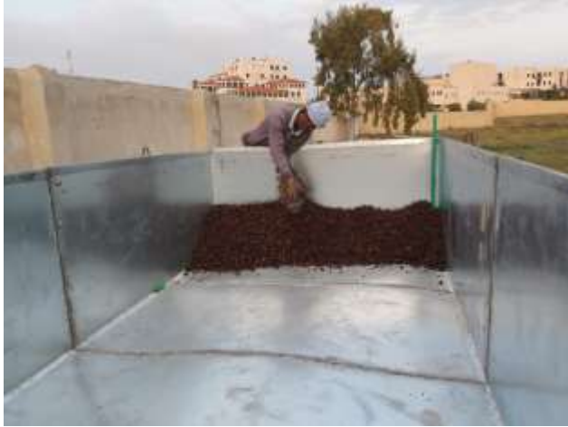
Figure A.7 Filter material distribution
