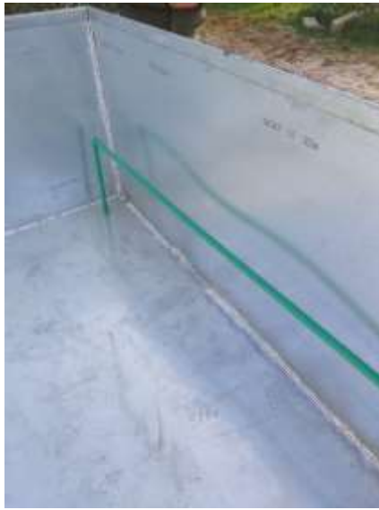
Figure A.6 Wetland plumping works
