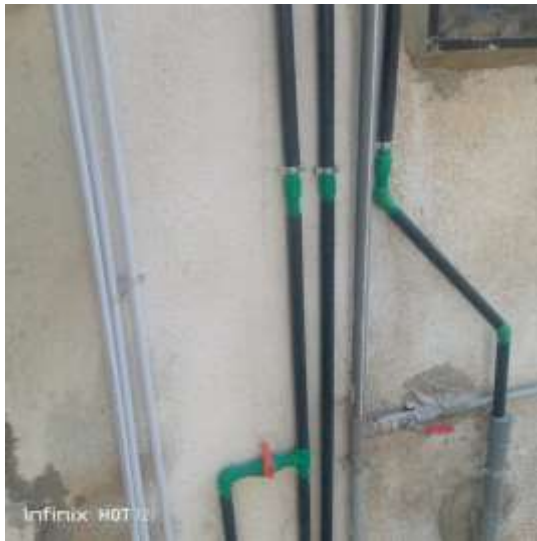
Figure A.9 Plumbing finishing works
