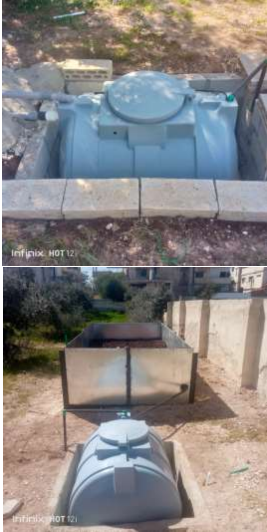
Figure A.11 Final system installation
