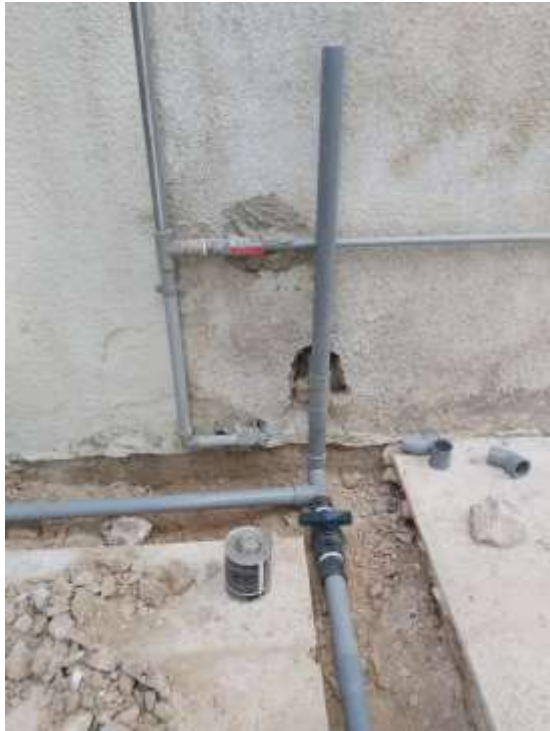
Figure A.2 Plumbing works
